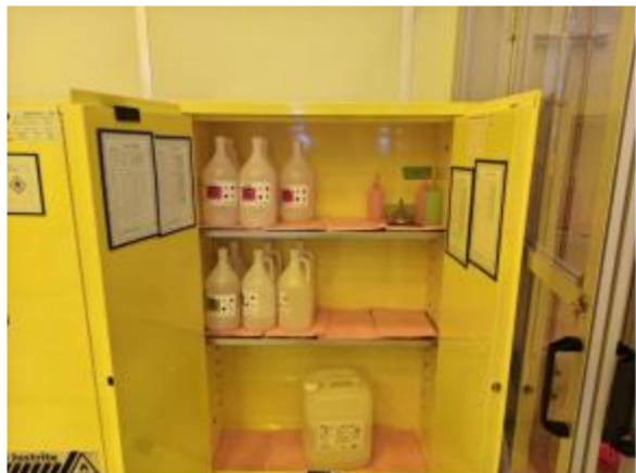
厂房内防爆柜
